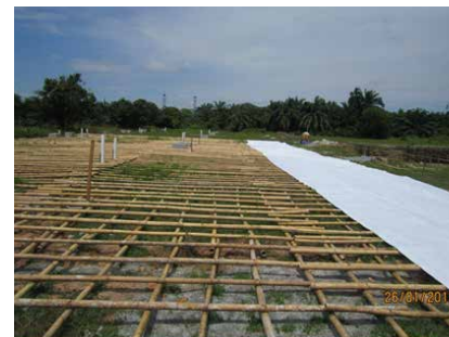
Plate 6 – Future houses to be supported on Bamboo-geotextile System over peaty soil and devoid footing – in progress
