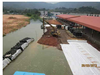
Plate 3 - Improvement of soft ground by Bamboo-geotextile System in progress
