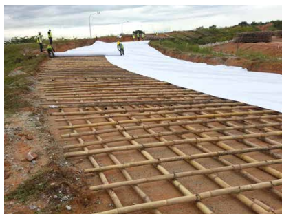
Plate 2 – Bamboo Grid Frame applied being overlaid by geotextile
