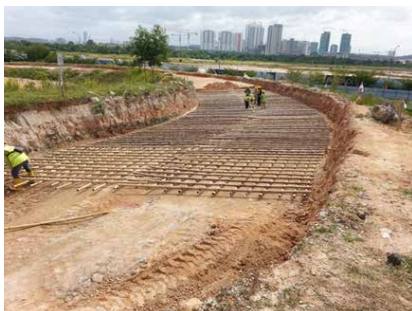
Plate 1 – Apply Bamboo Grid Frame System on clover-leaf Ramp for settlement arrestation
