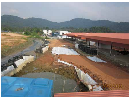
Plate 4 – Improvement of soft ground by Bamboo-geotextile System near completion
