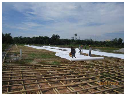
Plate 5 – Future houses to be supported on Bamboo-geotextile System over peaty soil and devoid footing – in progress
