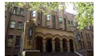
III / GSII Main Building.
