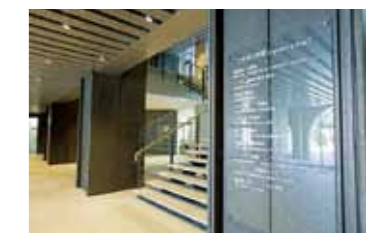
Engineering Building No.3, newly built in 2013.
