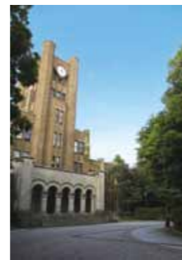
The clock tower, one of the landmarks of the Komaba Campus.
