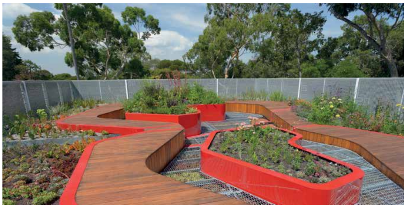
The demonstration green roof at Burnley
