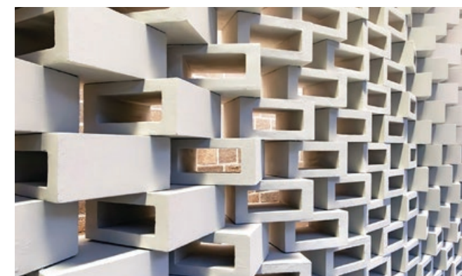
Eco-friendly construction materials made from recycled glass, or "eco-blocks", that can curb carbon emissions and turn waste into resources
